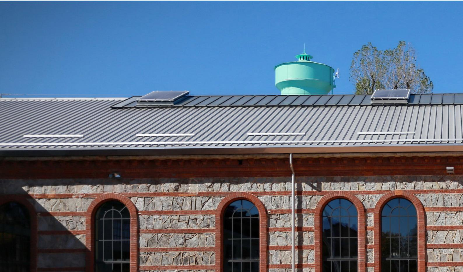
The different **ROOF** models constitute a complete system of pre-insulated monolithic metal panels, suitable for any type of roofing. The metal supports of the panels are made of metal sheets while the insulation is made of rigid polyurethane foam.
